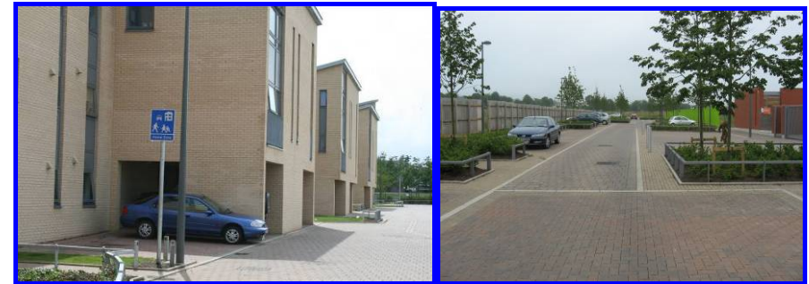
Figure 16. Pictures of the development at Wauchope Square
