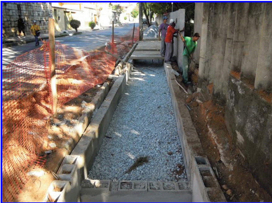
Demo filter drain in Belo Horizonte
