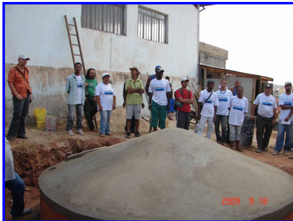
Installing a tank for rainwater harvesting
